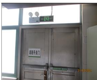
Photo of fire safety equipment Emergency exit with exit sign and emergency light.jpg
